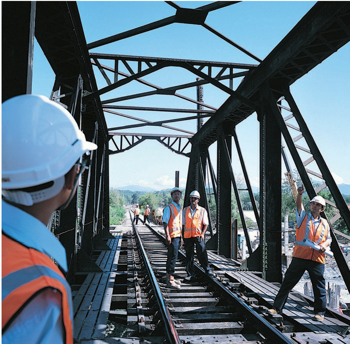
Electrified Double Track between Ipoh and Padang Besar Landasan Kereta Api Berkembar Elektrik Ipoh-Padang Besar
