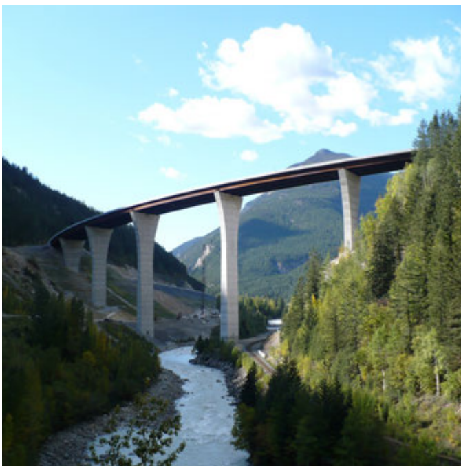
Kicking Horse Canyon Viaduct, Canada Jejambat Kicking Horse Canyon, Kanada
